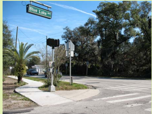
Motorists may encroach into the sidewalk area at the intersection of Blue Lake Avenue and S.R. 44
